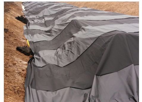
Contaminated Soil Windrow Cover
